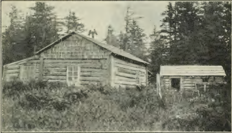
FIG. 11.—Living quarters and outbuildings constructed from native timber B24628
